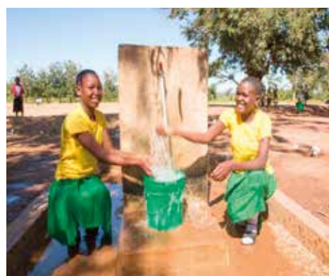
Plate 1.1 A newly installed water point at Kakora Primary School in Geita.
