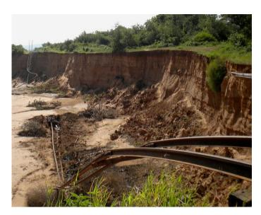
Plate 4. Severe flood damage to the CRL at Gulwe.
