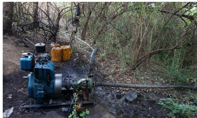
Diesel pump abstracting water from the Chongwe River
